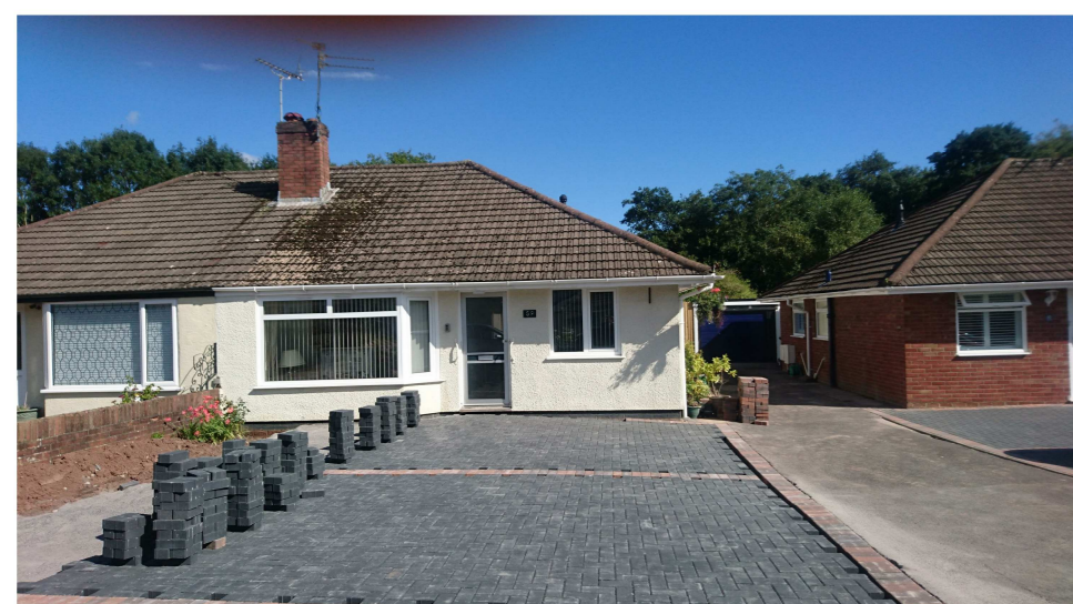
Existing Front Elevation Image 1
